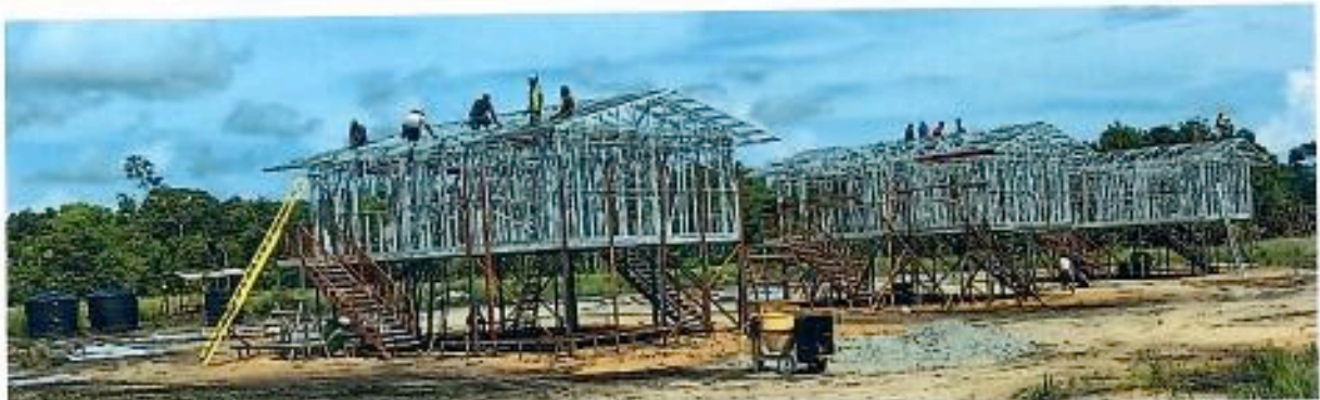
Three teachers houses' under construction at Edwaki High School in Telefomin District of West Sepik Province as part of the project obligations.
