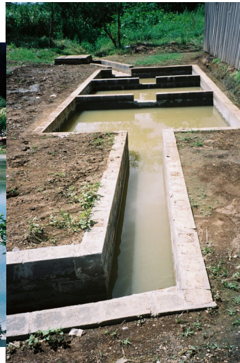
Left: Waste ponds behind the Cannery
